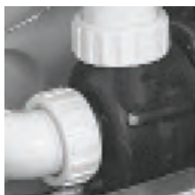
Vent air by slightly opening pump unions.
