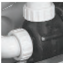
Vent air by slightly opening pump unions.
